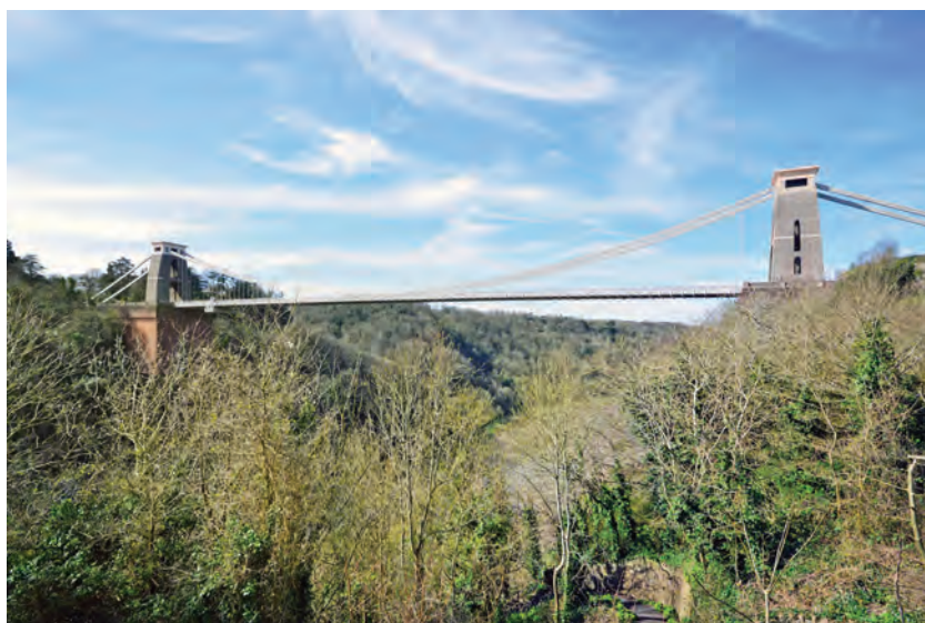
Clifton Suspension bridge seen from the south, with the Leigh Woods abutment under the left hand tower
